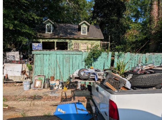
Property that may require nuisance abatement action.
