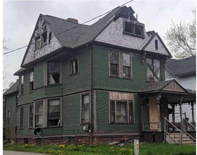
A fire damaged house in Bay City, MI. Photo Credit: Center for Community Progress
