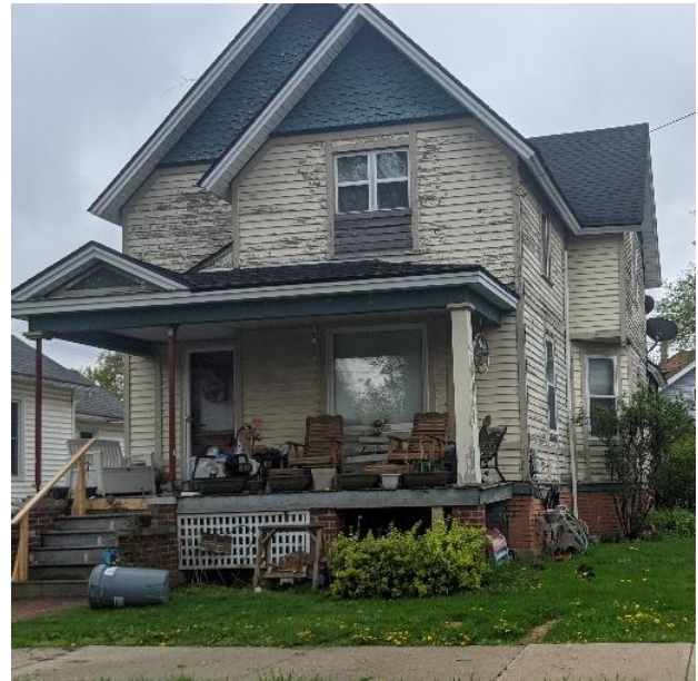
A home in below average condition in Bay City. Photo: Center for Community Progress
