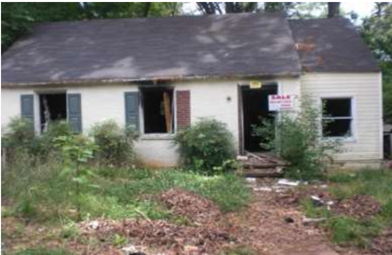
VACANT AND UNSECURED STRUCTURE
