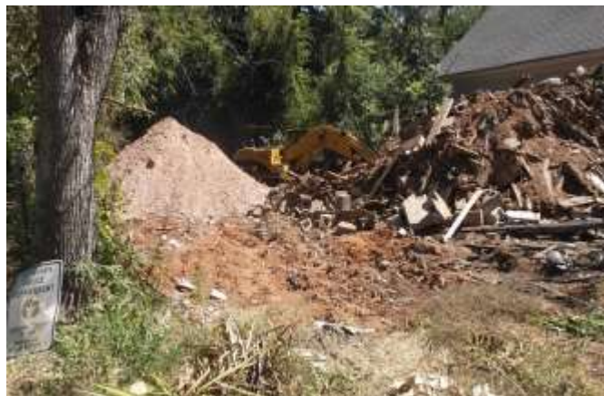
DEMOLITION OF 123 ATLANTA STREET
