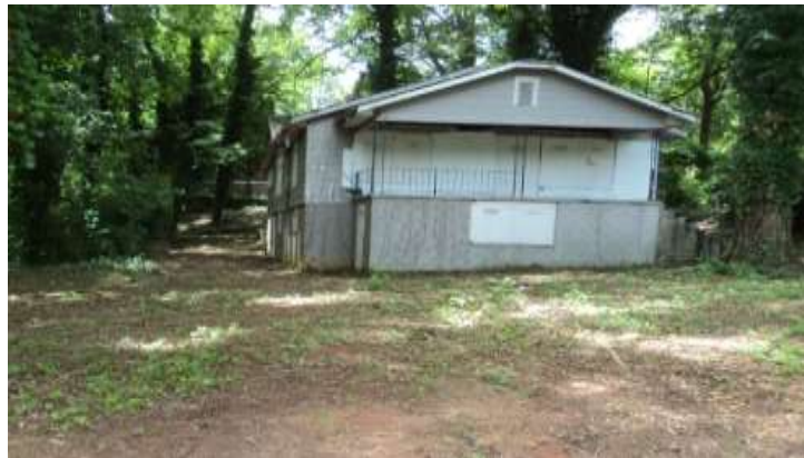
CLEANED AND CLOSED VACANT STRUCTURE
